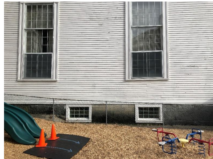
Sanctuary windows: Main floor and basement
