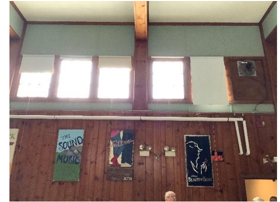
BE11 - Interior storms on these windows in the Parish Hall would add further insulation value.
