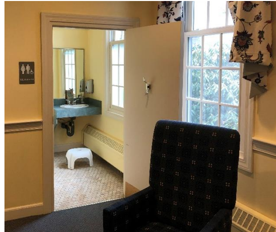
E2: Restroom candidate for occupancy sensor
