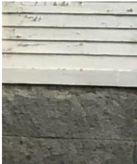
BE8 - Air sealing where the foundation meets the framing is important. Consider removing the trim board at the bottom of the siding then applying caulk, spray foam or a fluid-applied flashing.
