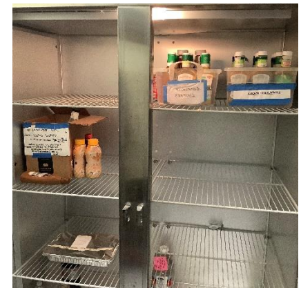
E6: Traulsen commercial refrigerator. Given how little is in here, could this be moved to the GE fridge and this one either turned off or the temperature turned up?
