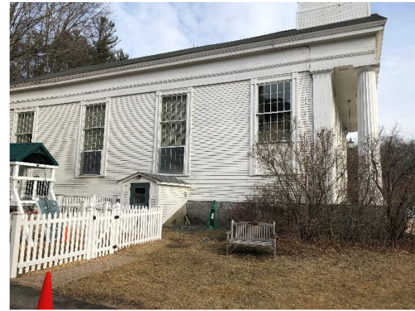
Southwest-facing Sanctuary Wall
