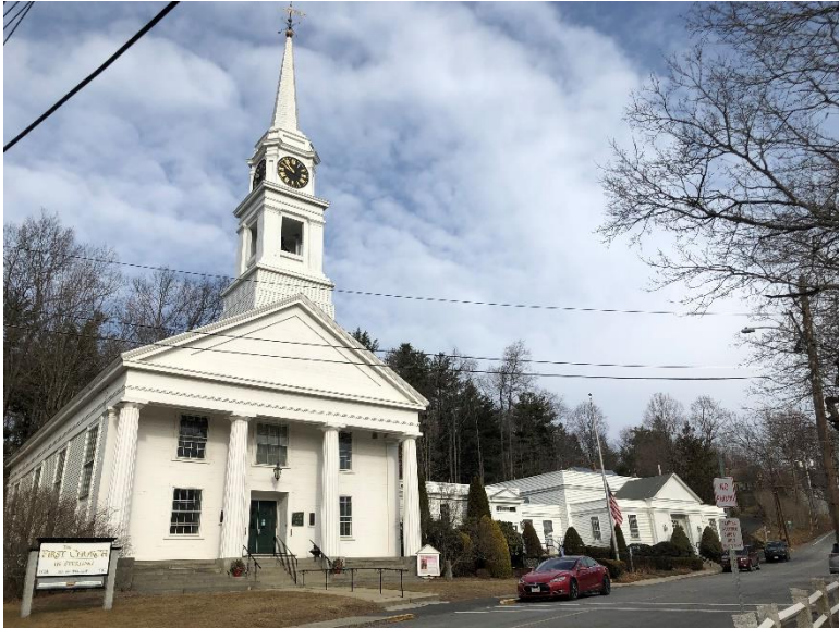
Street Level View from SE corner
